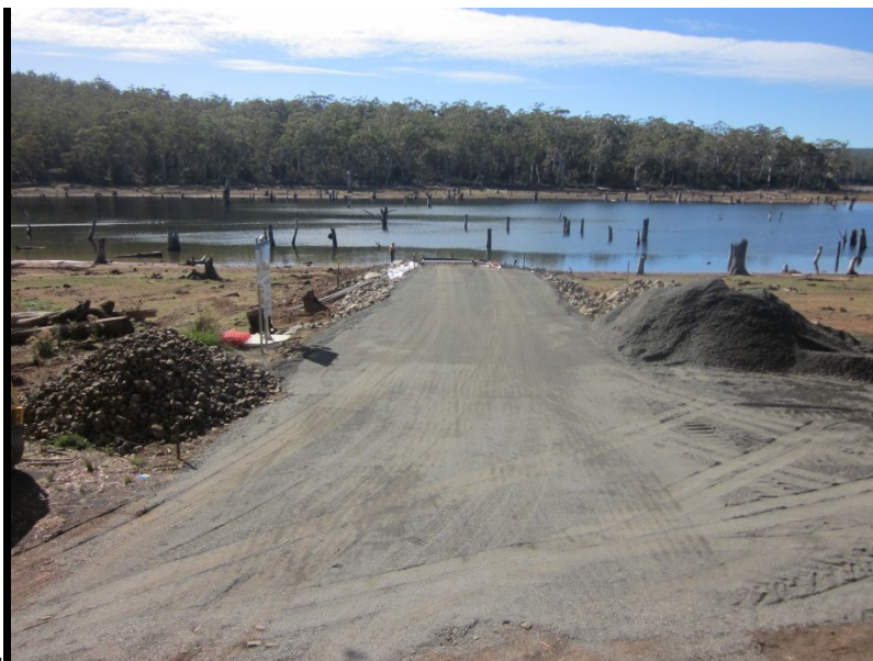
Lake Leake boat ramp upgrade – Photo Jim Caulfield
