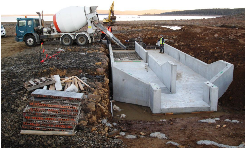
Fish trap under construction – Photo Neil Morrow
